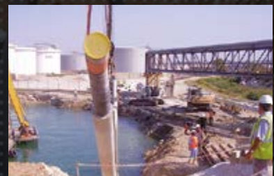
Laying of pipe in a sea inlet towards an oil deposit
